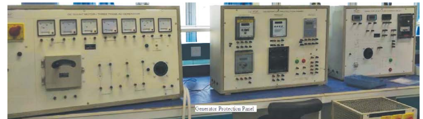
Power System & Protection Lab :- Numerical Relay Development Environment (NRDC) for Research on Power System Protection ,ETAP-Software
