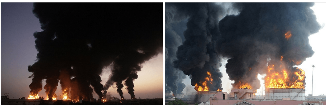
Fig. 1.1 Fire explosion at oil depot Jaipur, Rajasthan (Mail online, 1 November 2009)
